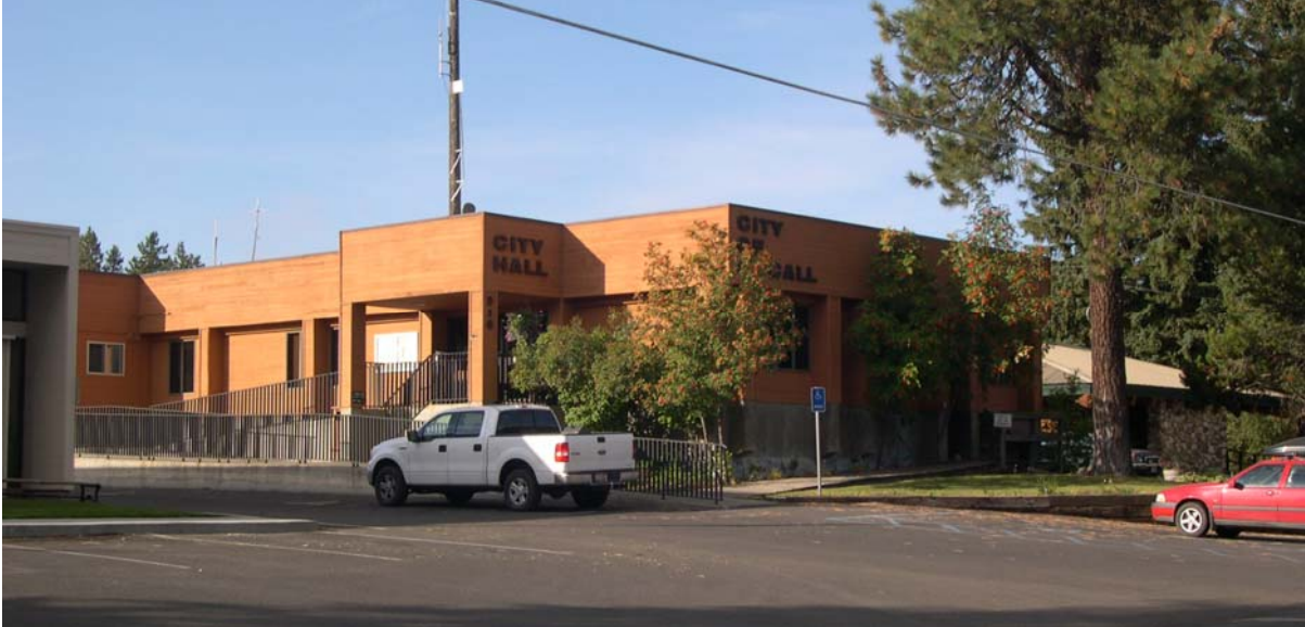
Existing City Hall Building
